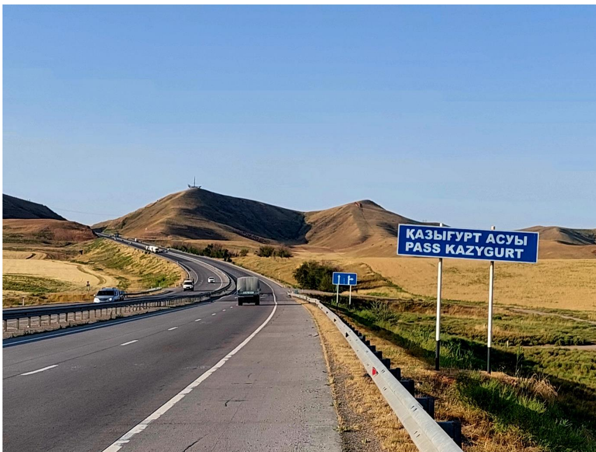
Shymkent - Tashkent Road
